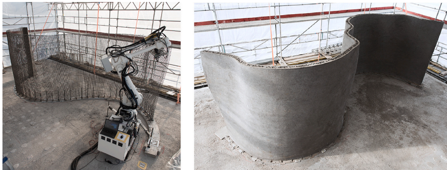
Fig. 6. Example of mold-less shaping with internal matrix (credit: NCCR Digital Fabrication, ETH Zurich).
