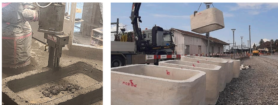
Fig. 4. Example of shotcrete 3D printing (credit: Mobbot SA).
