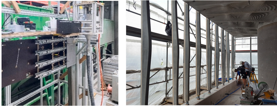
Fig. 5. Example of concrete slip-forming (credit: NCCR Digital Fabrication, ETH Zurich).
