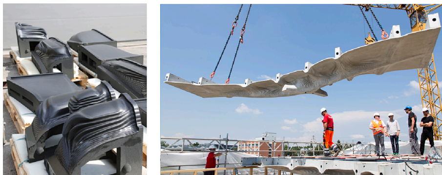
Fig. 3. Example of binder-jet printed formwork (credit: digital building technologies, ETH Zurich).
